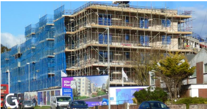
West block under construction
